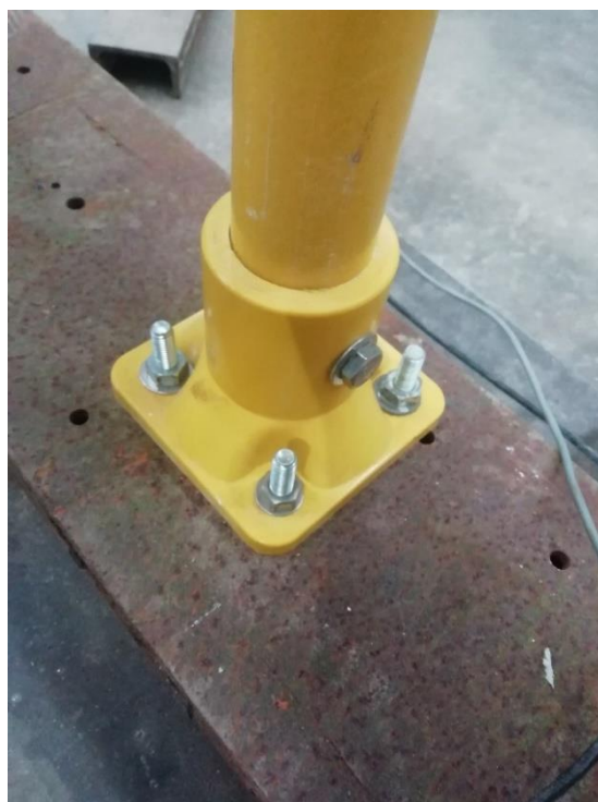
Plate 1 – Typical Feet Fixings
